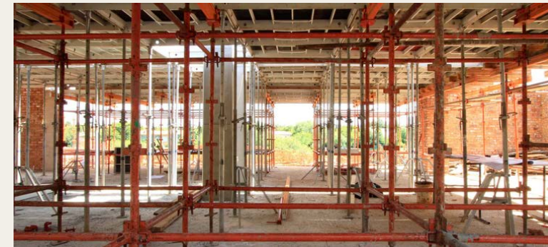
SCAFFOLDING PROPPING & DECKING
